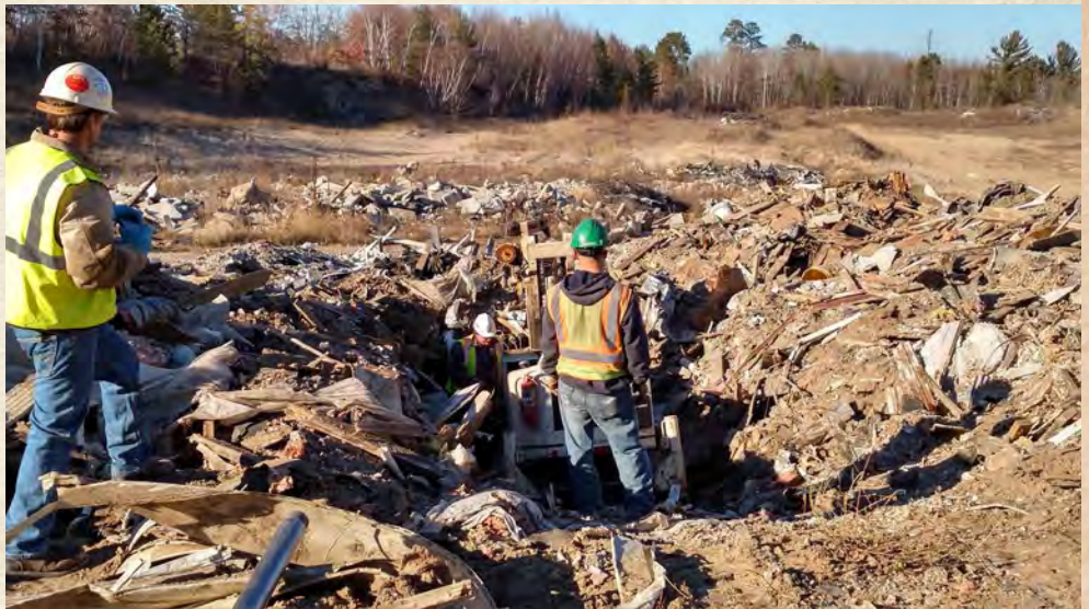
Tom, Joe and Jake of Environmental Troubleshooters Inc. drilling for soil samples at the illegal dumping area.
